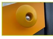
11-The Coat Hook is made of polypropylene.
