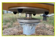
**9- The Balancing board** is fitted to a galvanized steel post, diameter 114 mm. A ball and socket joint ensures ease of movement.
